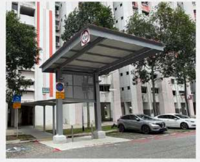
Upgrading of Drop-Off Point at Blk 102 Jurong East St 13
