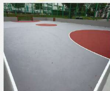
New Hard Court Flooring at Blk 334 Clementi Ave 2
