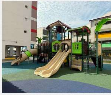
Upgrading of Playground at Blk 468 / 473 Jurong West St 41
